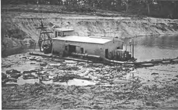
Dredge mining at Raymond Terrace, similar to that planned by CRA for our area, except that in the Wimmera there are deep clay layers above the sand
