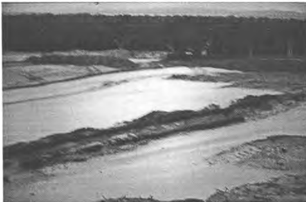
First stage of rehabilitation at Raymond Terrace. Topsoil ready to be spread
